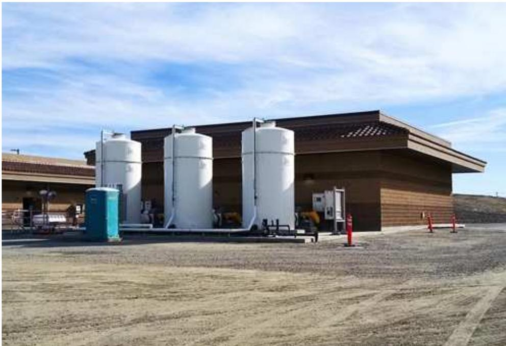
*BioAir's project in Coachella, Calif., features three EcoFilter<sup>®</sup> EF82 units, designed to control odor from a headworks facility. Courtesy: BioAir.*
