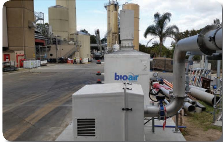
Once installed in the Tooheys brewery in August of 2014, le Roux said the EcoPure and EcoCarb technologies immediately began removing more than 99.9 percent of hydrogen sulfide (H<sub>2</sub>S) odors and the majority of organic odors from the airstreams of the wastewater facilities without using any chemicals.
