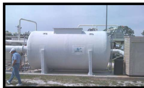
2,000 cfm Horizontal Bioscrubber
