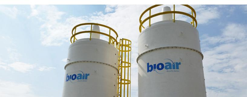
Biofilters have proved somewhat successful in eliminating odors and **regulated emissions**, but the persistent reliance on them is often based on the misguided use of Empty Bed Residence Time (EBRT) as a design parameter, a practice which is **not backed up by rigorous scientific study**.
